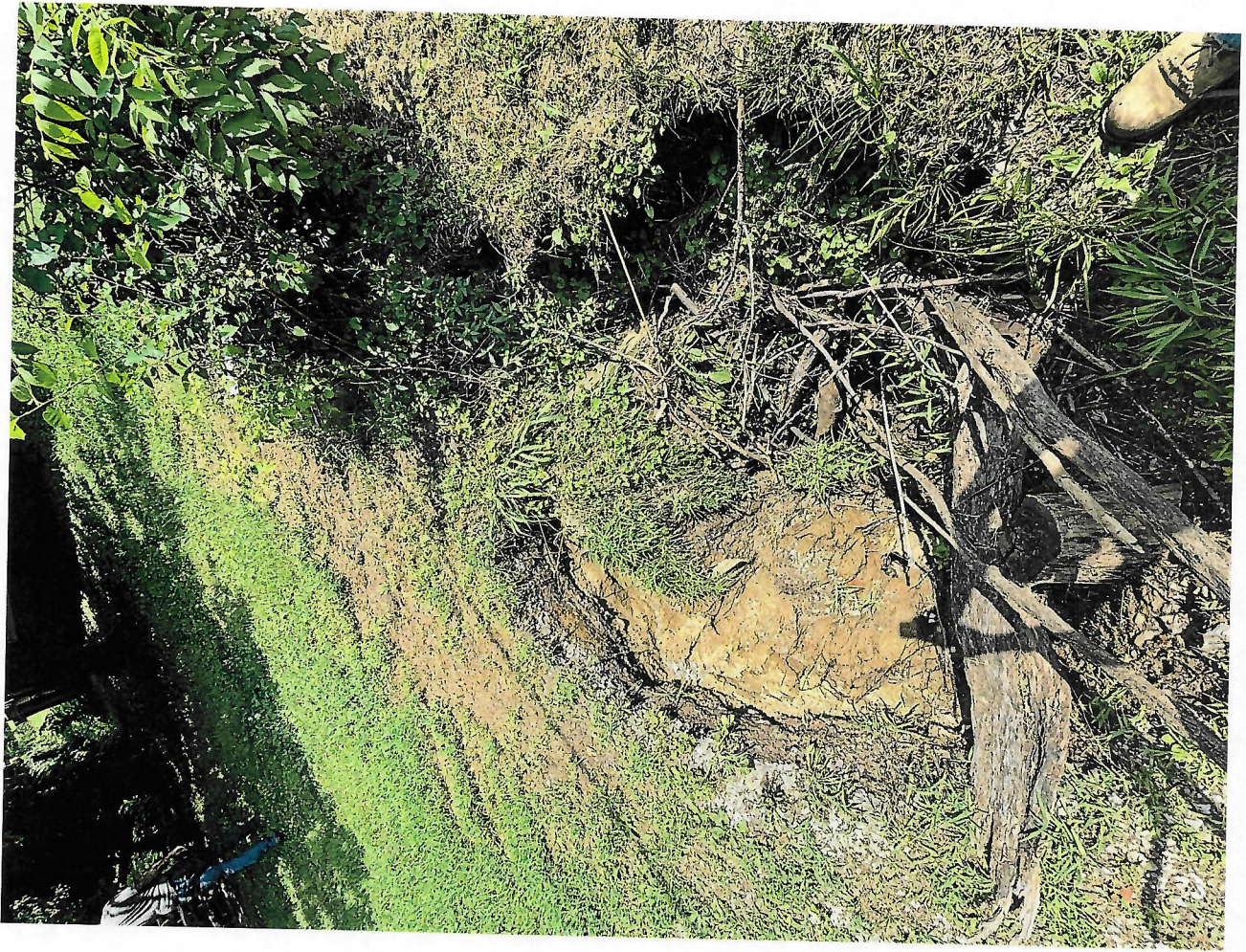
Sink hole on S East St where the existing driveway culvert is failing.
