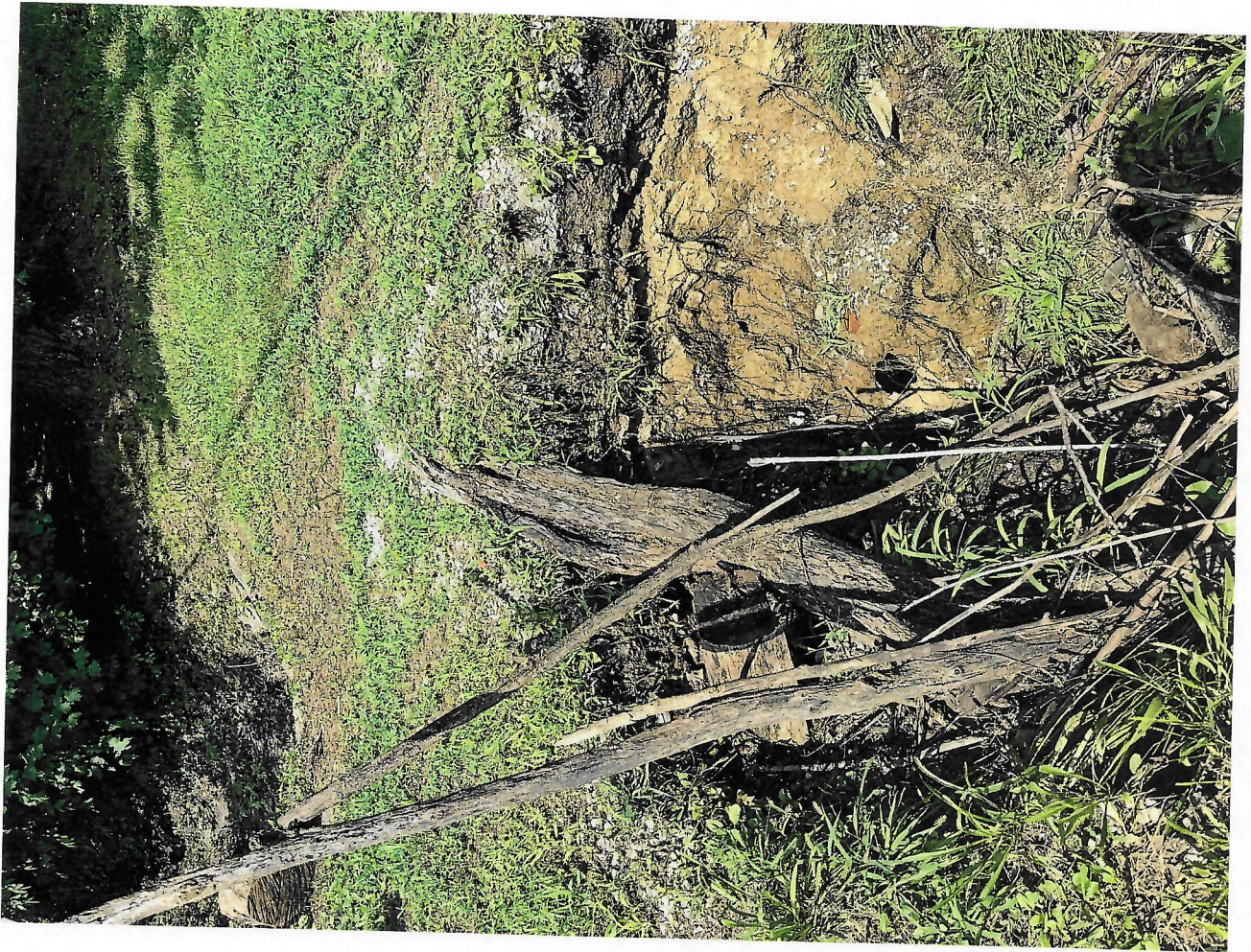
This picture has a better view of the galvanized culvert that is causing the sink hole.
