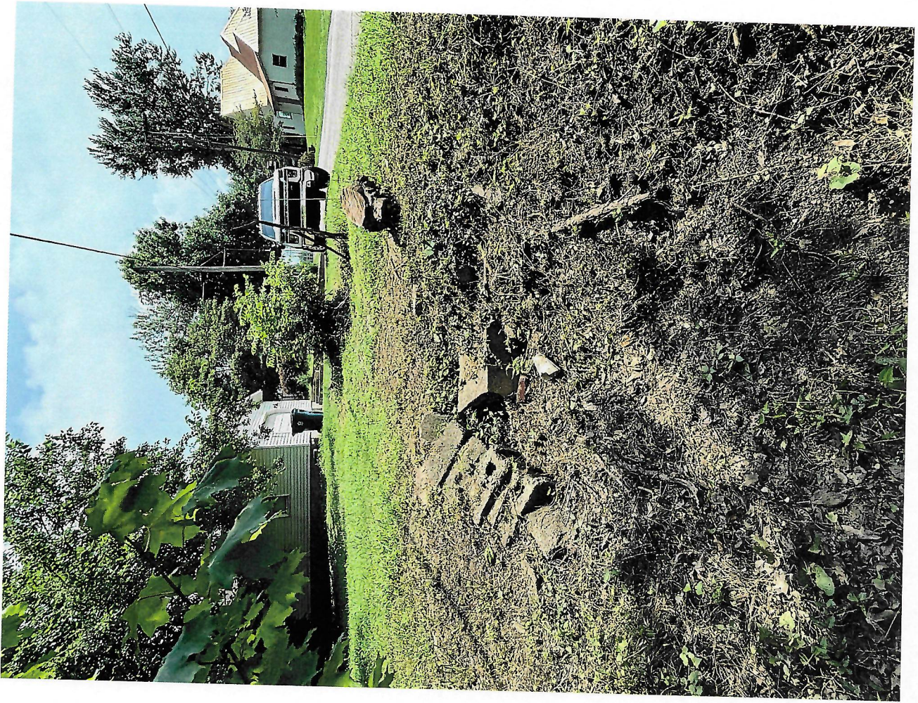
This is the current culvert inlet on the northern side of the home owners driveway. The new culvert or tee will have rip rap placed around the inlet.
